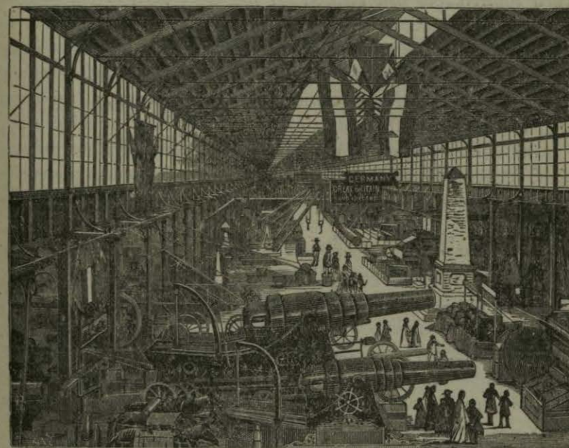
INTERIOR VIEW OF MACHINERY HALL.
