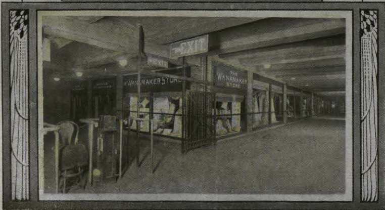
View of Elevators and Fire-door. Chestnut Street Entrance. Subway Entrance.
