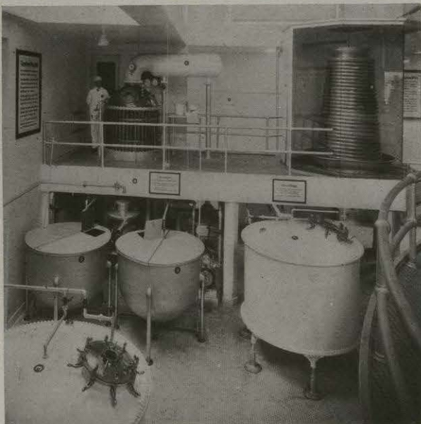
Milk plant, showing clarifier, vacuum pan, cooler, and holding tank.
