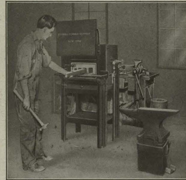
Fig. 86. — Oil furnace with water-jacketed front.
