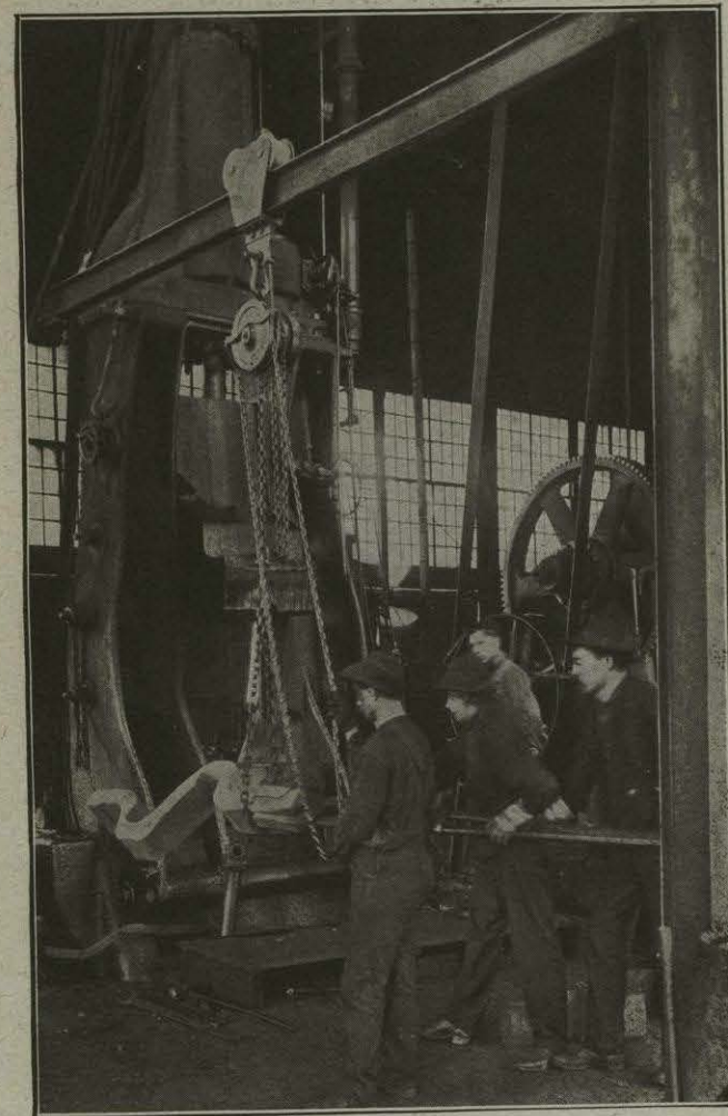
FIG. 64.—Removing partially forged 400-pound crank-shaft.
