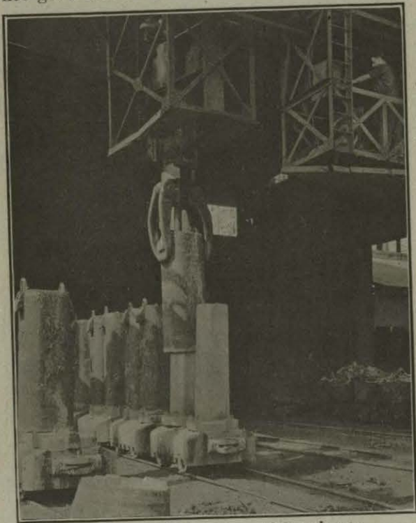
FIG. 13. — Stripping the mold from ingots.
