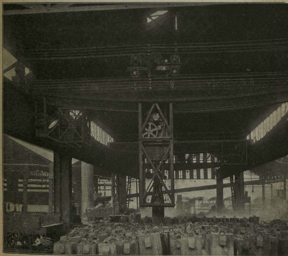
Fig. 58.—Guided Ingot Stripper.
