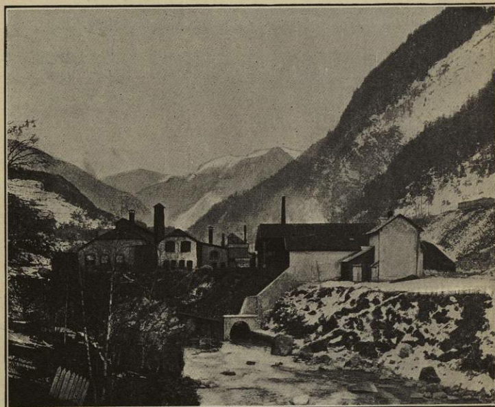
FIG. 23.—General View of the Steel Works at La Praz, France.
