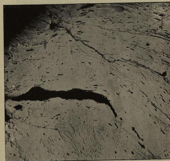
Fig. 99.—Section of a boiler plate cut from near a rivet hole distorted and crushed. The hole was enlarged by chiselling. The plate gave way when being tested under water pressure at a point close to where the section was cut. Note the cracks represented by continuous black lines in the figure. \times 50 .
