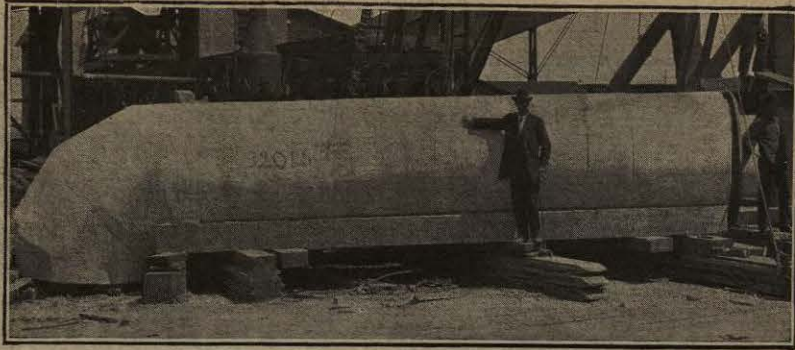
54 inch Intake Pipe for Public Service Corporation of New Jersey. Marion, N. J., Power Station
