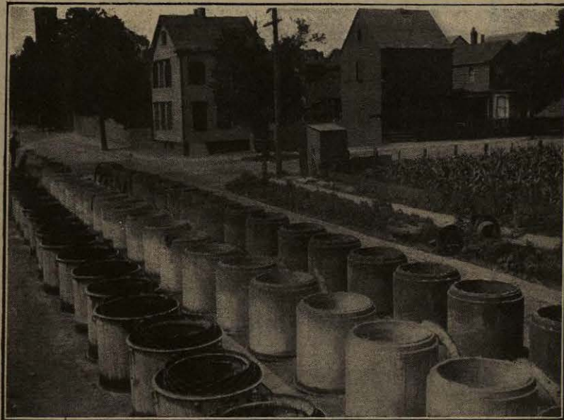
Making Pipe for Newark, N. J., Sewers
