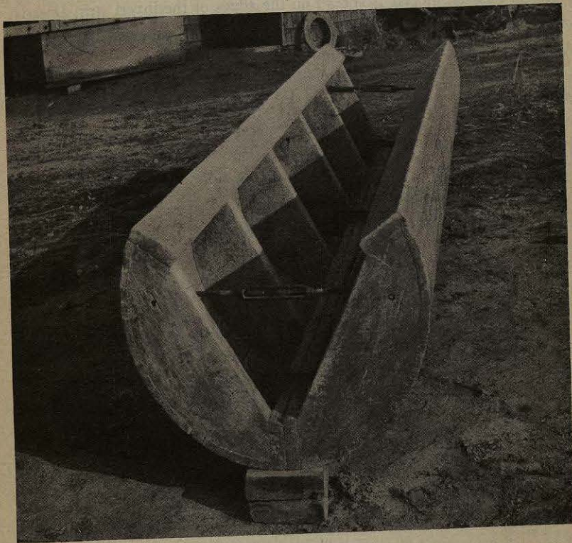
FIG. 224. — Center for Invert of 30-inch Sewer at Medford, Mass. (See p. 688.)
