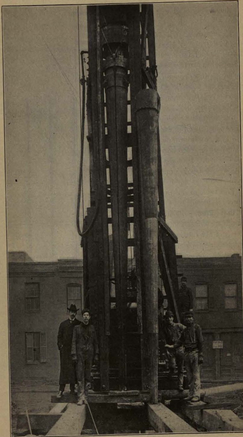
FIG. 207. — Cores for Concrete Piles. (See p. 650.)
