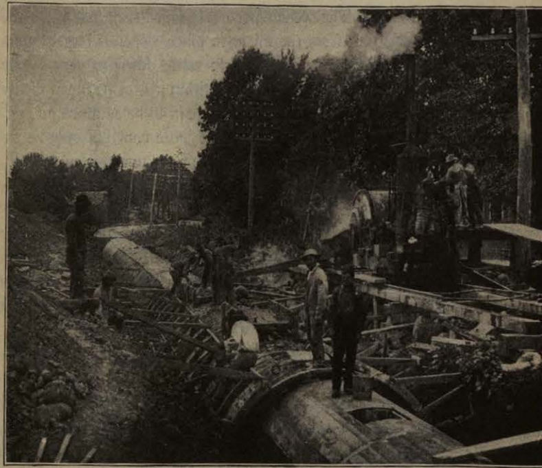
FIG. 97.—Depositing Concrete through a Trough. (See p. 278.)
