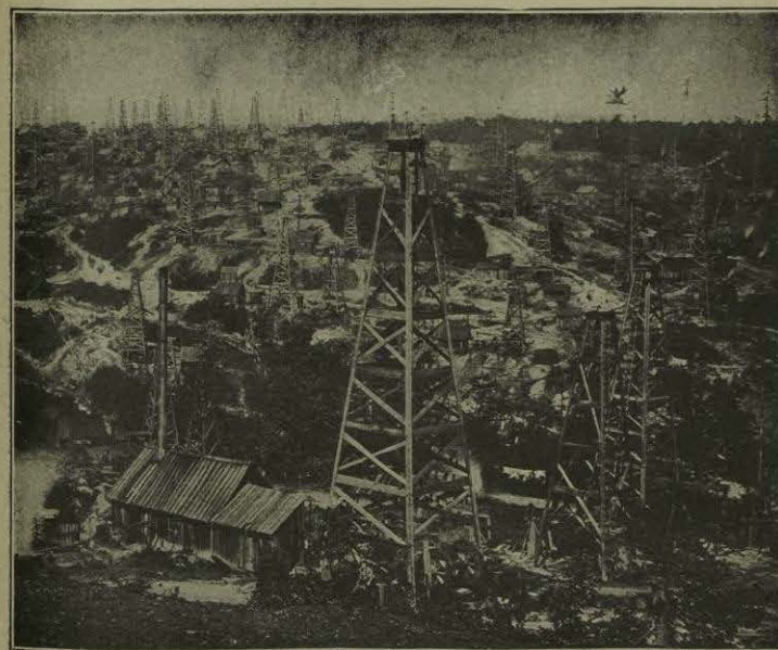
FIG. 542. — Each of these derricks marks the site of a boring for oil at Tidioute, Pa., in 1870. From these wells large amounts of oil were obtained.
