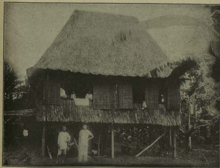
FIG. 527. — Thatched house in the Philippine Islands, needed for protection from sun and rain, not cold. It is raised above the ground to avoid dampness and to prevent the entrance of animal pests, which are very troublesome.
