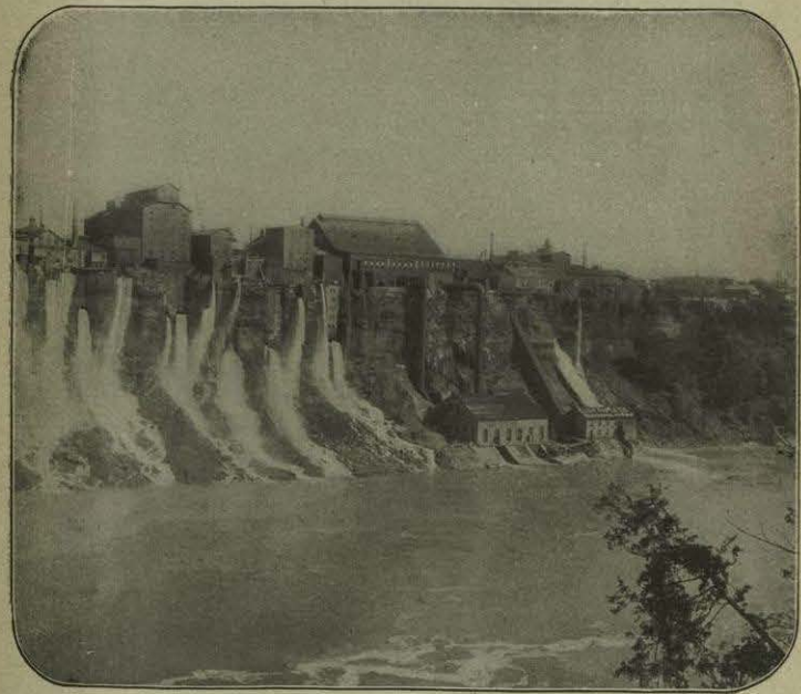
FIG. 484. — The water escaping here is a small portion of that used for power at Niagara Falls. Yet only a very minute portion of the enormous power available is now used.
