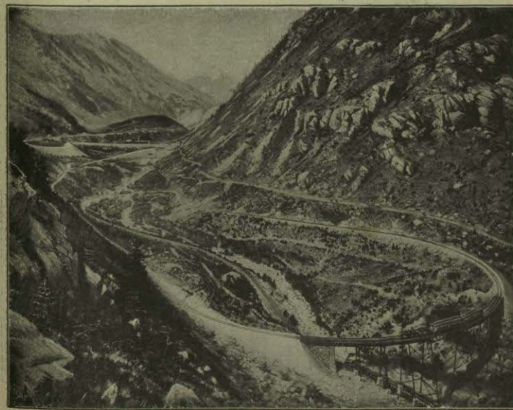
FIG. 471. — A railway line crossing the Rocky Mountains near Georgetown, Colo.
