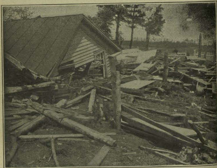
FIG. 422. — Destruction done by the tornado at Mt. Morris (Fig. 420). In the roof of the upper figure, notice the laths driven through boards by the force of the wind.
