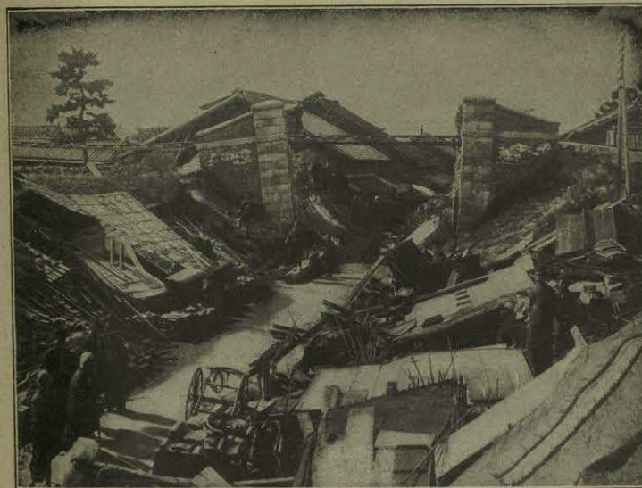
FIG. 241. — Destruction caused by the Japanese earthquake of 1891 (Fig. 239). All this damage was done to houses that were built very lightly and thus able to withstand ordinary earthquake shocks.
