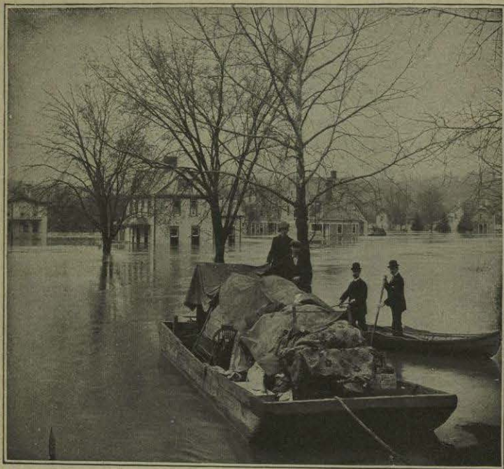
FIG. 99.—The Ohio River in flood near Parkersburg, West Va. Notice that the water rises to the first-story windows.
