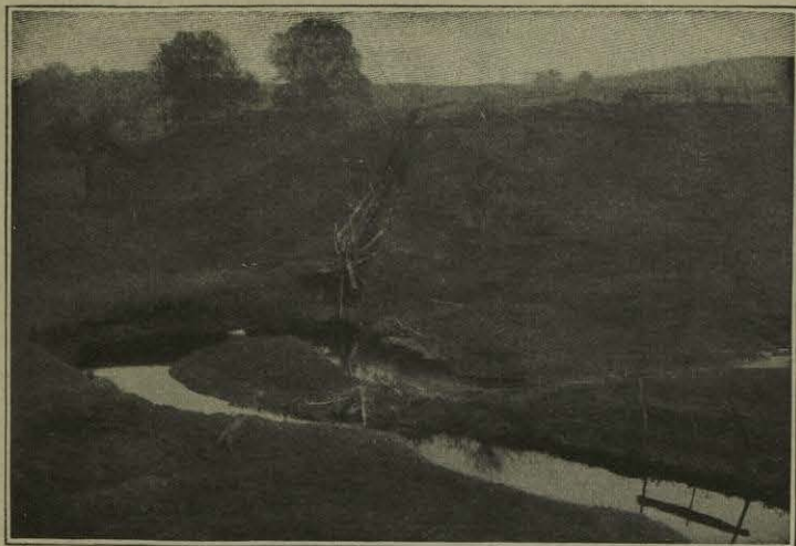
FIG. 94.—A small ox-bow curve in a meadow brook. A cut-off has been started, but brush was put in to stop it from continuing. (L. O. Towne, Haverhill, Mass., Photographer.)
